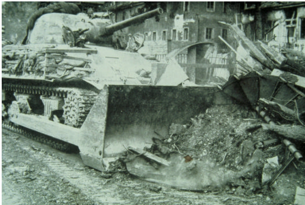
Fig. 13. Sherman tankdozer. Reprinted courtesy of CARL.
